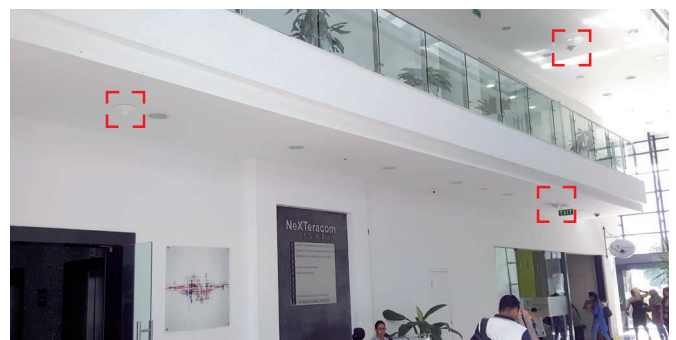
Lobby of Nexteracom office building with Kathrein antennas
